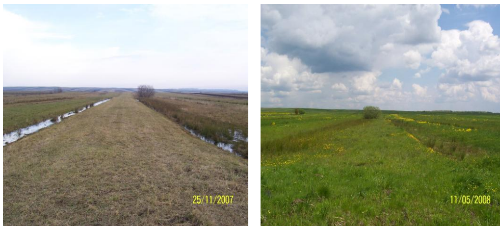
Photo 1 Water stagnation and the onset of humidity seeking vegetation on channels
