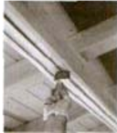
Fig.7.26 Carbon fiber plates strengthening on a wooden beam
